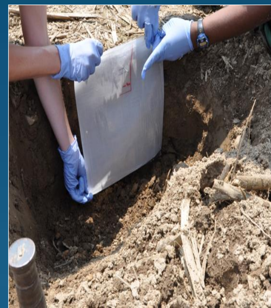
Installing resin sheets
