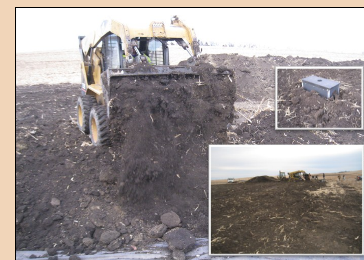
6. Completing the installation by backfilling the topsoil .
