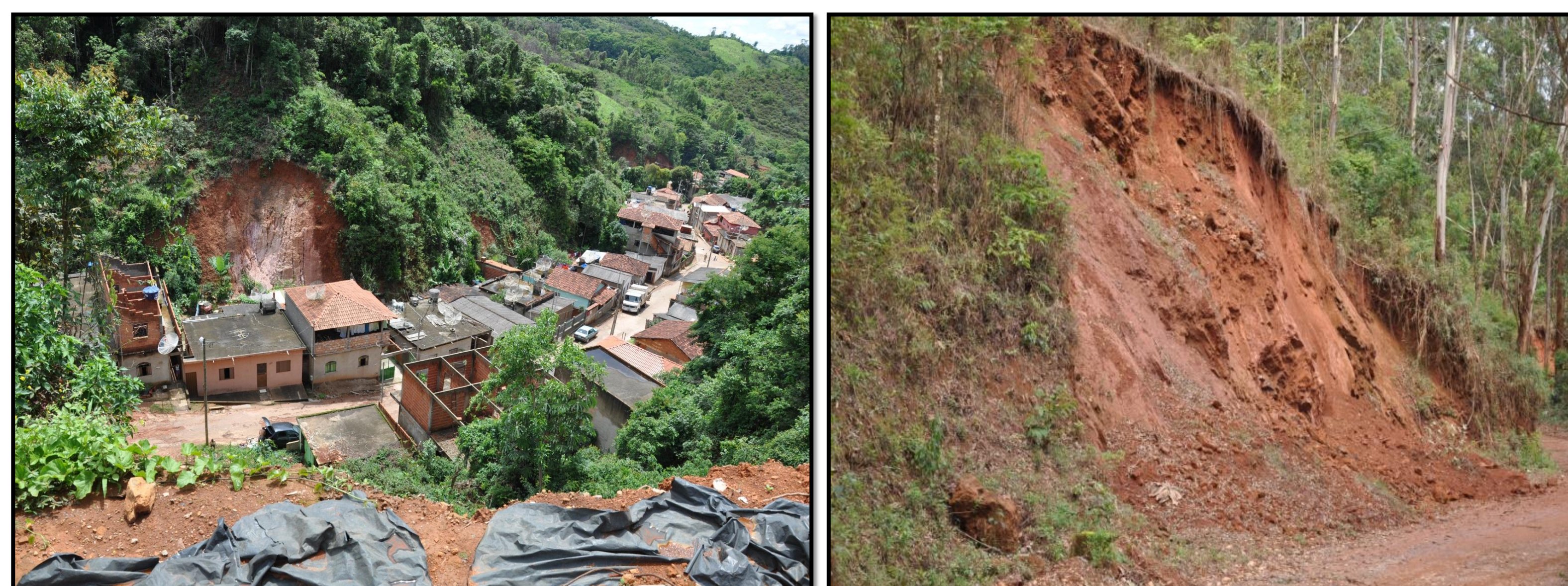
Figure 2: Landslide in Piranga County, Minas Gerais, Brazil
