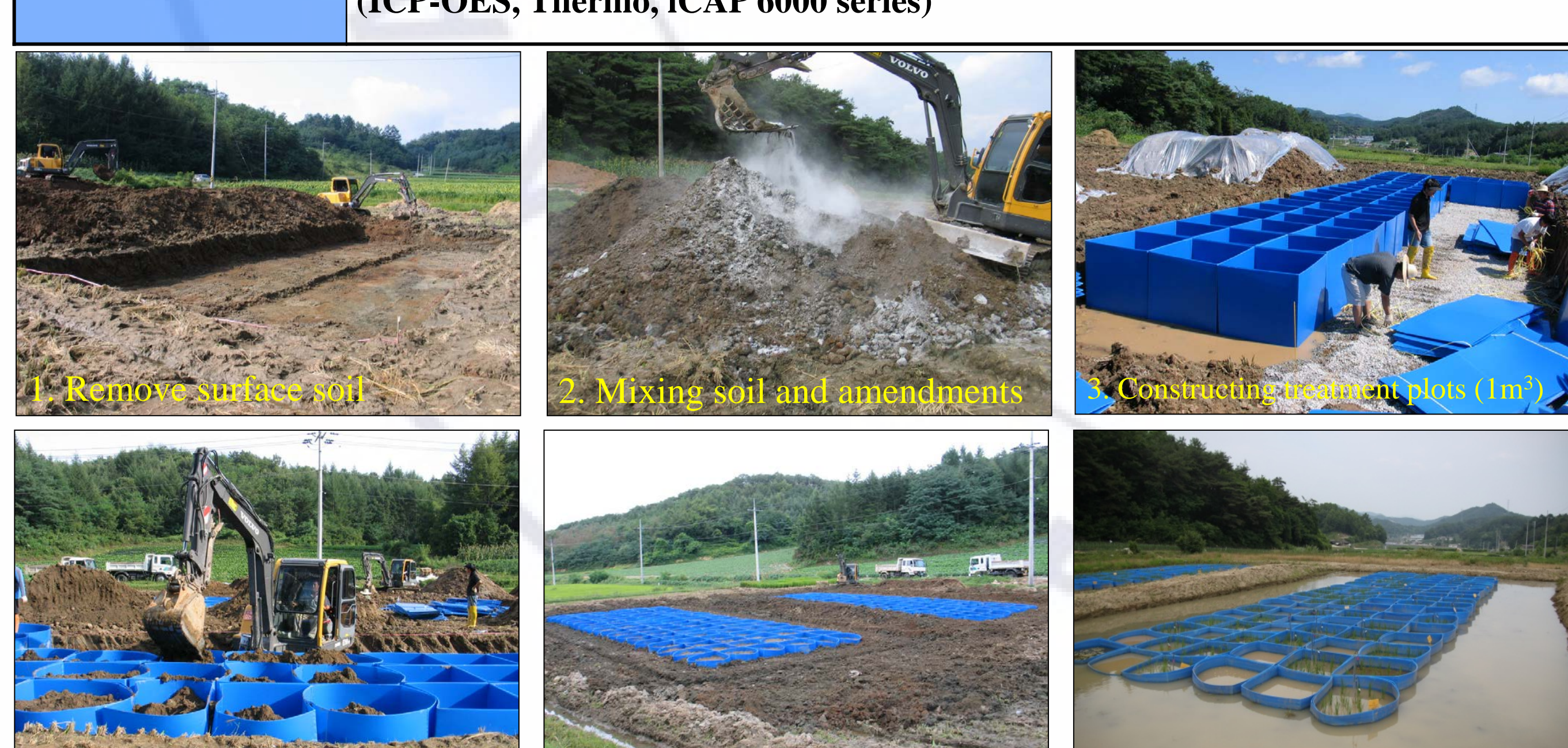
Figure 1. Process for constructing treatment plots
